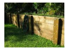
NOTE: TYPICAL DETAIL ONLY. ALL WALLS WHICH FORM PART OF DRAINAGE WORKS MUST BE BUILT AS DETAILED BY THE HYDRAULIC ENGINEER. ALL WALLS EXCEEDING 800mm SHALL BE OF NO TIMBER CONSTRUCTION MATERIALS, CONSTRUCTION DETAILS TO BE PROVIDED BY A QUALIFIED ENGINEER. INSTALL WALL TO SUIT SITE LEVELS AND TO MANUFACTURE'S SPECIFICATION.
